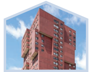
BAYVIEW TOWERS, CONNECTICUT (BEFORE)
