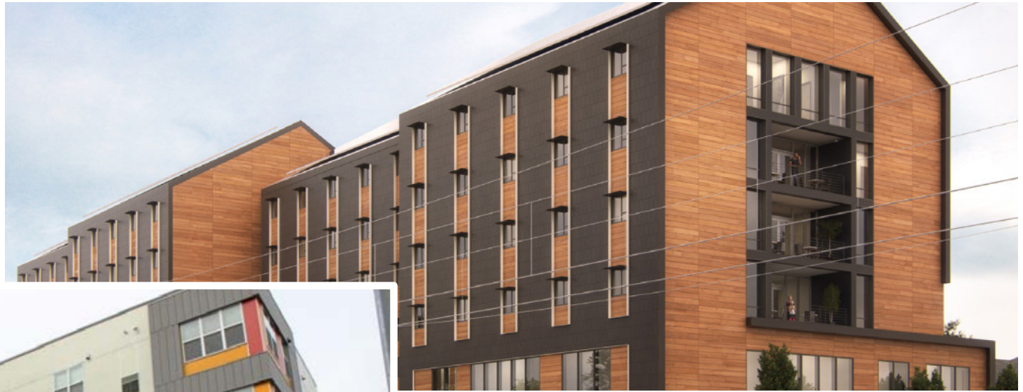
Blackburn Building, Portland Central City Concern & Housing is Health Alliance
