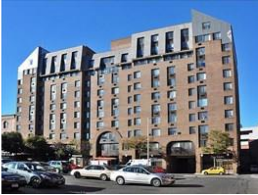
Exchange Place Tower, Waterbury, Conn.
