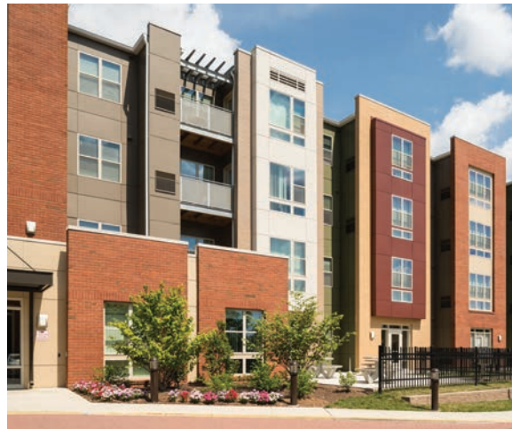
AFTER NEW CONSTRUCTION
