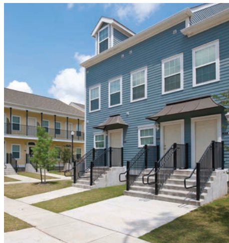
AFTER NEW CONSTRUCTION
